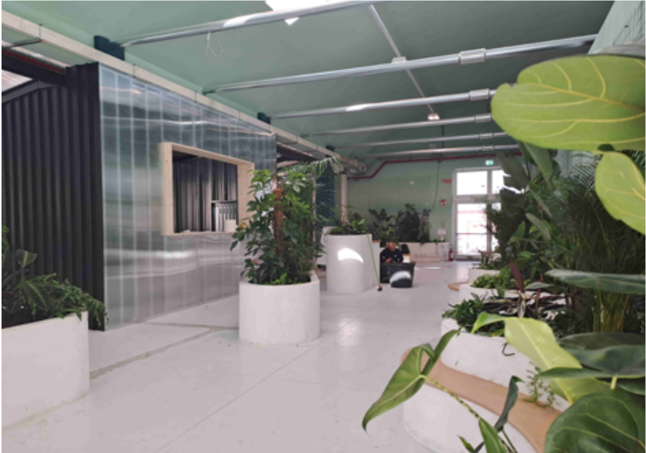
Fig.9 - Internal view of the City Market at the Macrolotto Zero - construction phase (credits: PNAT)
